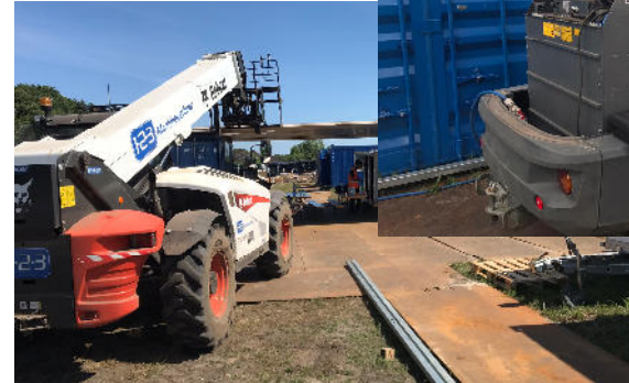
more electric machines on site
