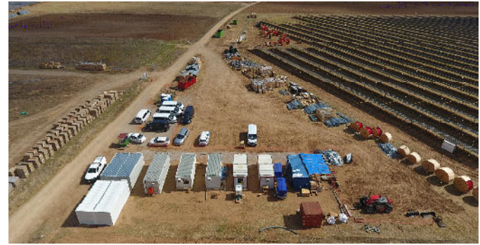
site with office and working containers
