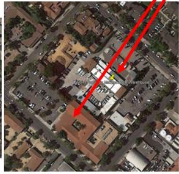
District Food Warehouse & District Office
